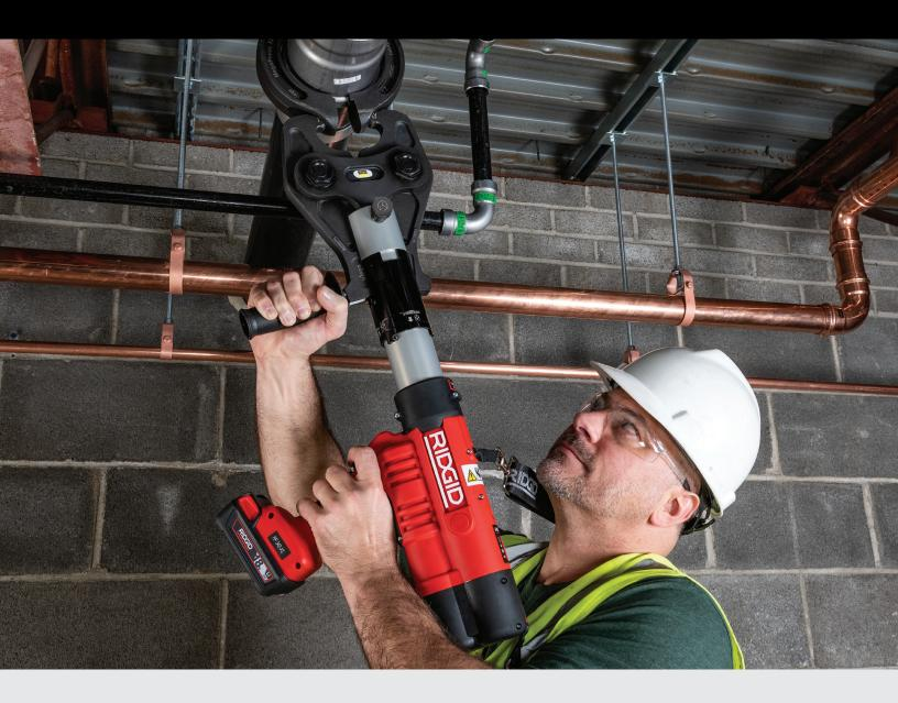
The RP 342-XL is the first ever RIDGID® press tool that works on any size and material pipe. From ½" PEX all the way up to 4" carbon steel\*, one tool can press it all. It also works with the full line of RIDGID Standard 32kN attachments including fan favorites like StrutSlayr® and PressSnap®. Its compact design and versatile applications make it the tool you want for every job.
